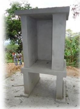
The 5,000-gallon tank has been repaired and is ready to use as the cistern for the pump. They have also finished constructing the cement box which will safely house the pump's control panel (pictured to the left of the tank). A pump technician has reviewed the structures and provided final recommendations to prepare for pump installation in the near future.
