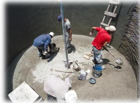
Construction has begun on the new, 10,000-gallon tank which will serve for centrally treating and storing the water for distribution to the community. The foreman works alongside local masons from Buena Vista to build the watertight structure from bricks, rebar, and cement.
