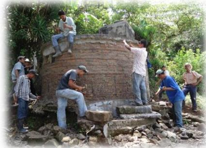
Community members prepare the current tank for repairs by removing the old cement seal.
