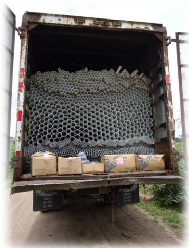
A truck delivers over 2,000 PVC pipes and several boxes of piping accessories to Buena Vista.
