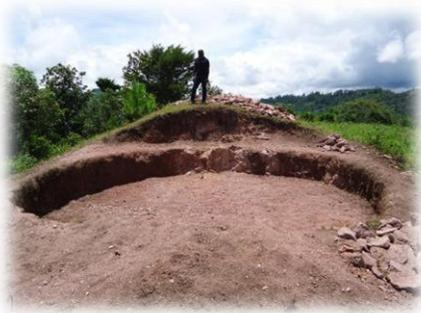
Work groups from Buena Vista leveled the land of the new tank site and dug the area for the tank's foundation.
